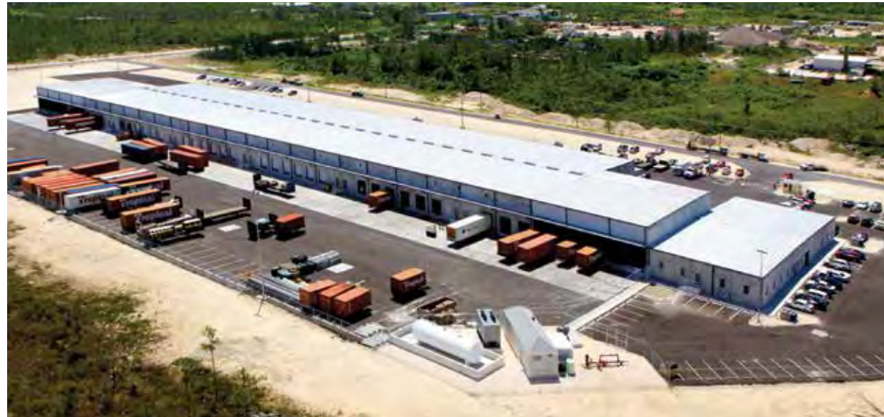
Arawak Development Corporation, Nassau, Bahamas, inland container handling facility
