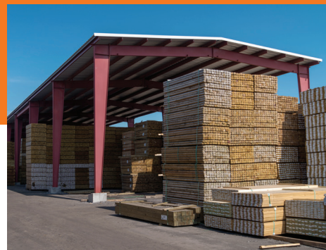
51' wide shed designed to allow enclosing in the future
