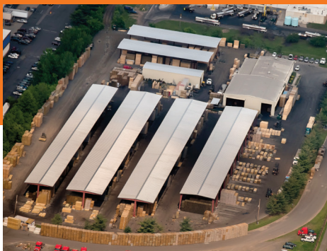
Reconfigured site with over 90,000 sq. ft. of new sheds
